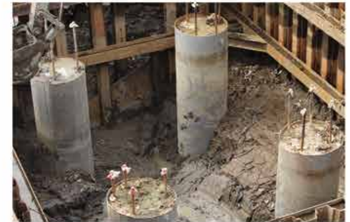
Boring pile for bridge foundation
