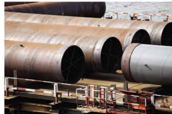
Steel pipe pile foundation for bridge construction
