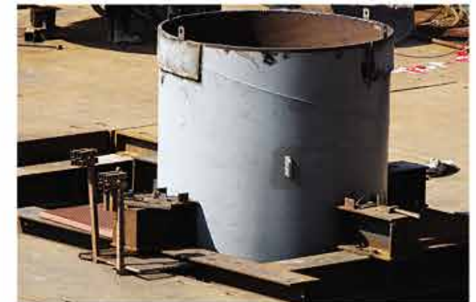
Steel pipe pile foundation for bridge construction
