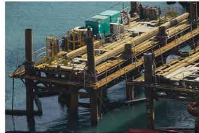
Tin Tunnel project
