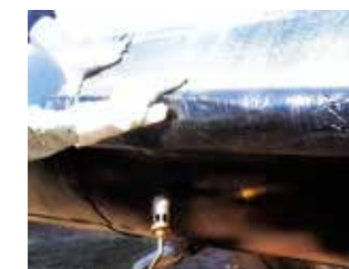
Coal Tar Tape Application
